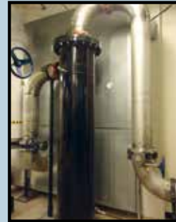
Protecting heat exchangers, Nevada USA
