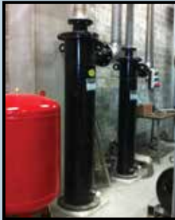
Cleaning chilled water, Axima Belgium
